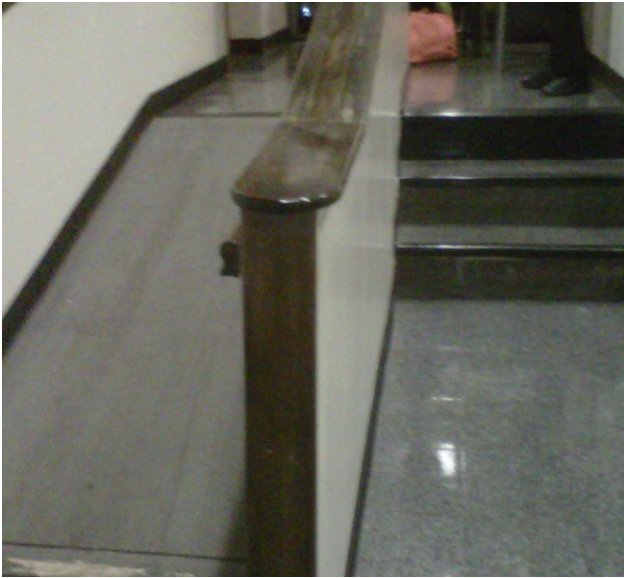
NYU Carlyle- steep ramp with one handrail
