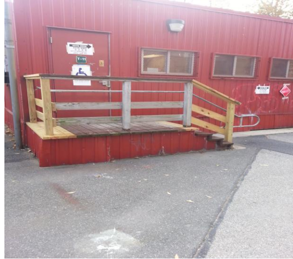
PS 214, Brooklyn, NY – Confusing signage at main entrance. Accessibility sign with no directional information.
