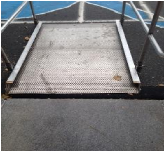
122 Henry St. NY - temporary ramp with gap between the landing.
