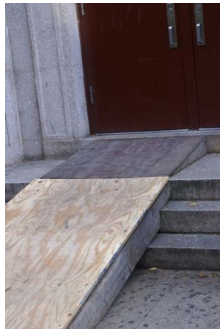
At Seward Park High School (Manhattan) there are two ramps. The ramp's handrails at the main entrance jut into and narrow the width of the doorway. If someone's wheelchair is too large to get through this doorway (pictured above), there is a separate entrance that has a dangerous ramp without handrails, edge protection or level landing at the top (pictured left). It leads to a locked door without a monitor.
